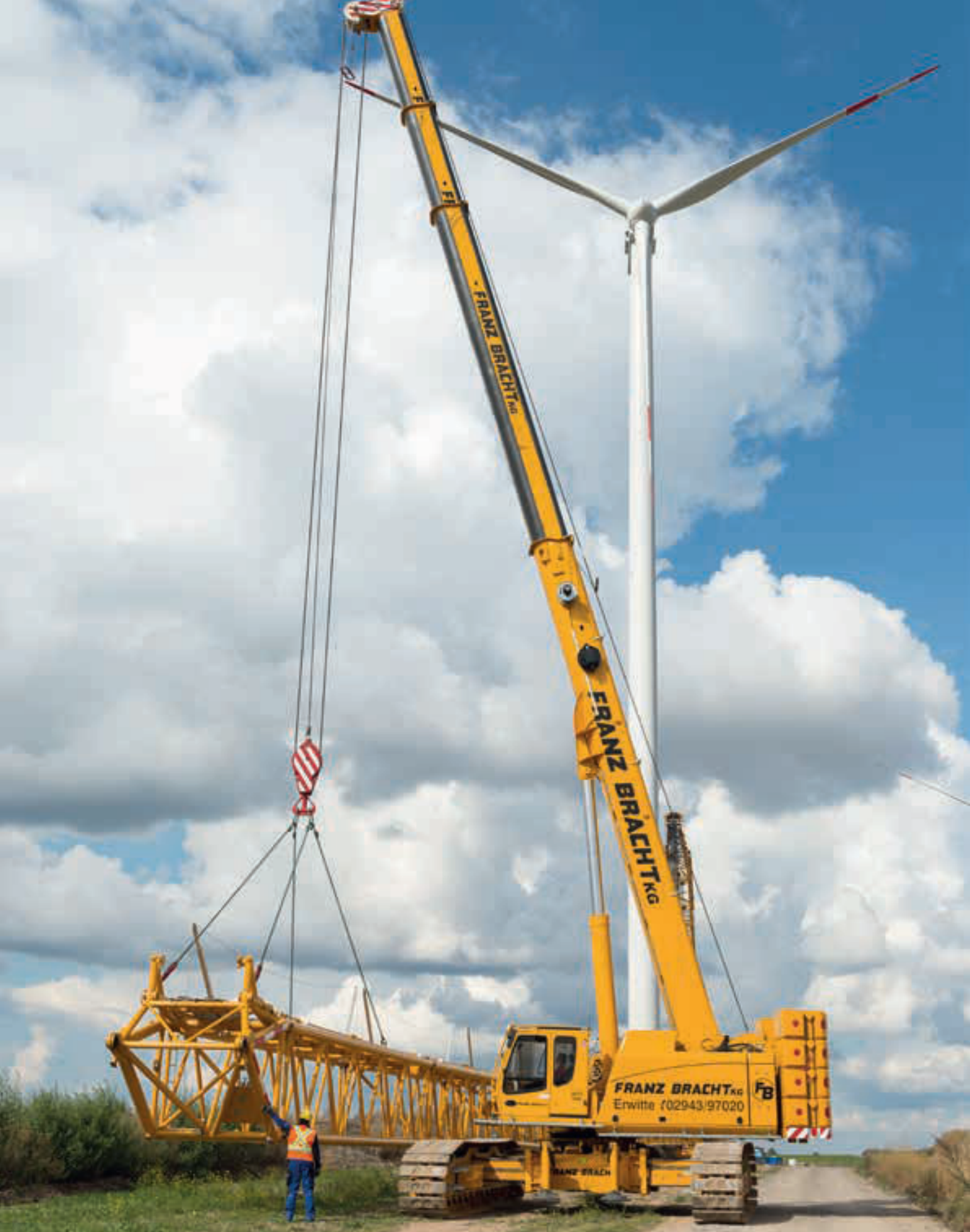
6113 R - used as a flexible service crane in wind energy; Germany
