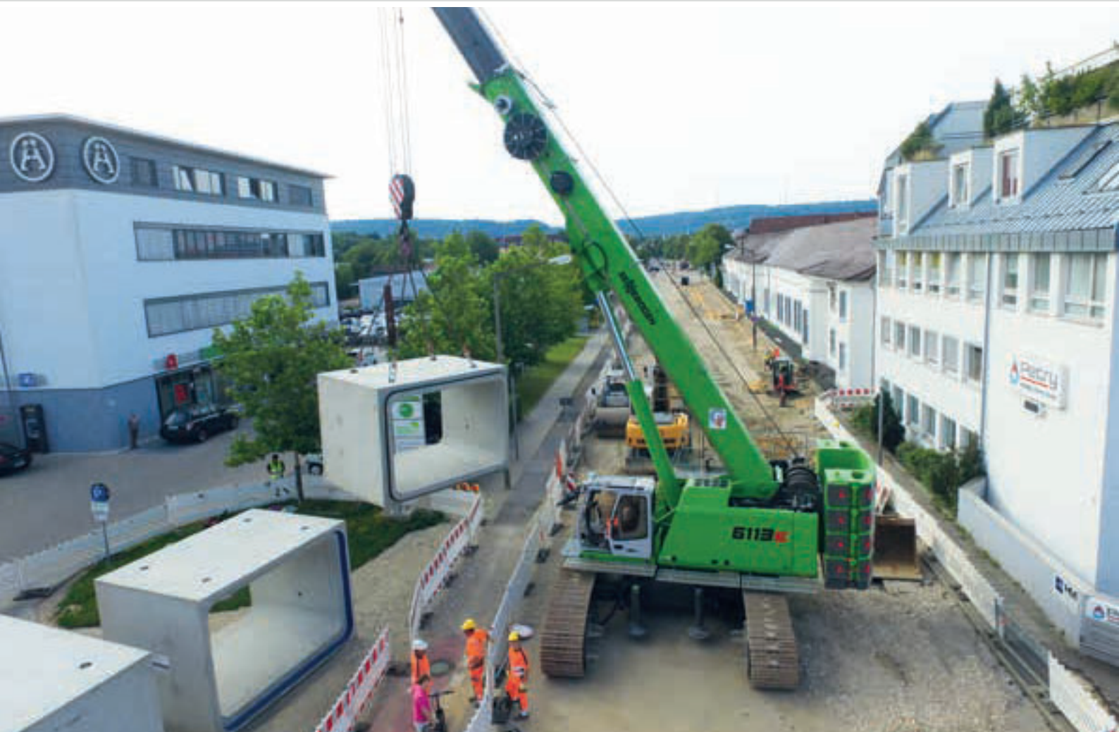
6113 R - high stability on any site surface with Star-Lifter broad gauge chassis; Germany
